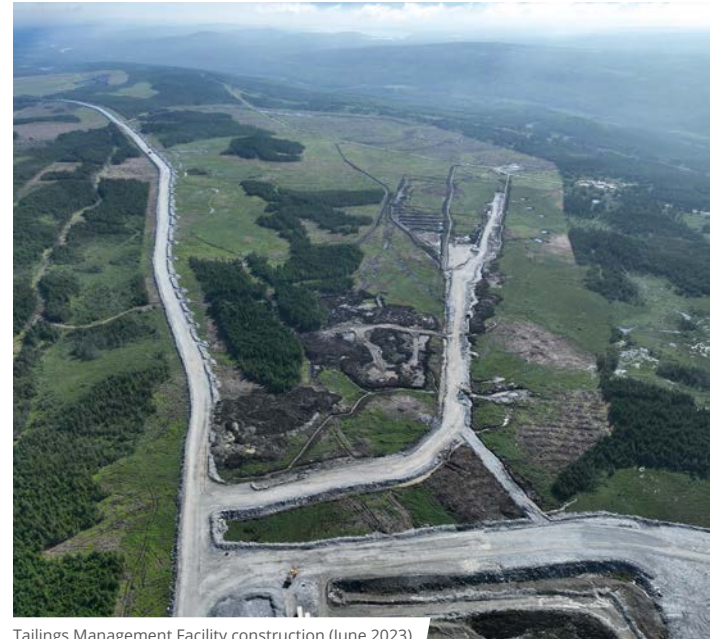
Tailings Management Facility construction (June 2023)
